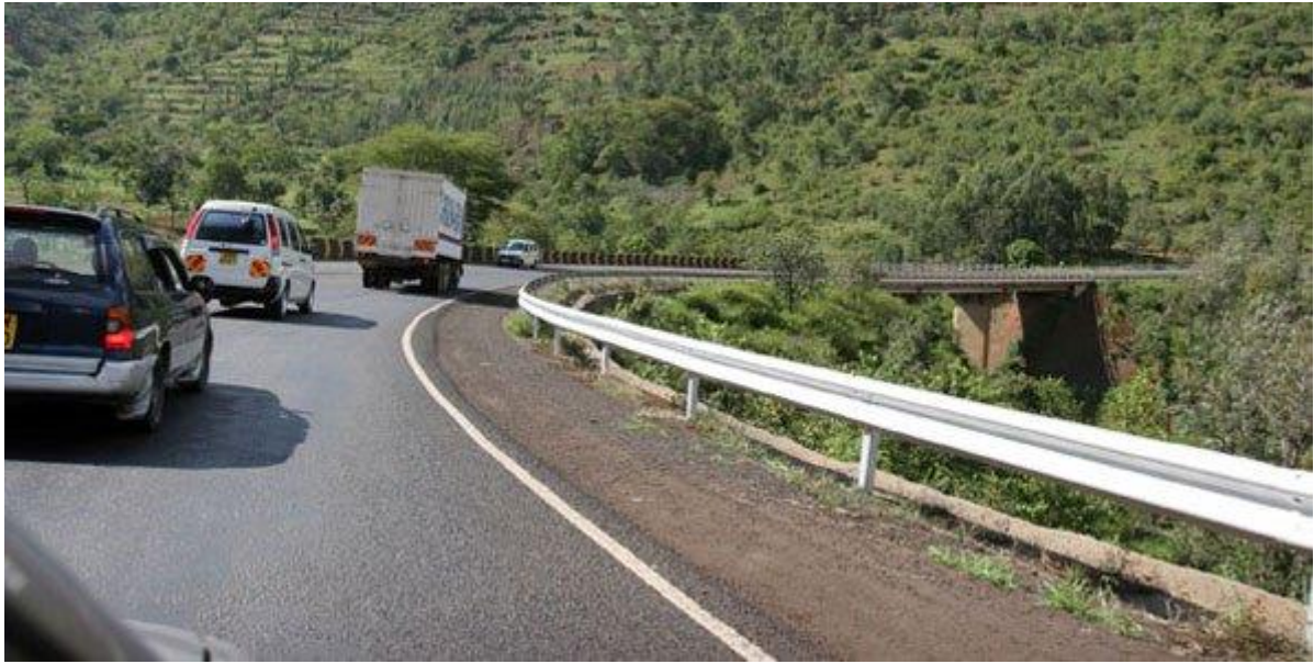
Picture 1: Nithi Bridge
