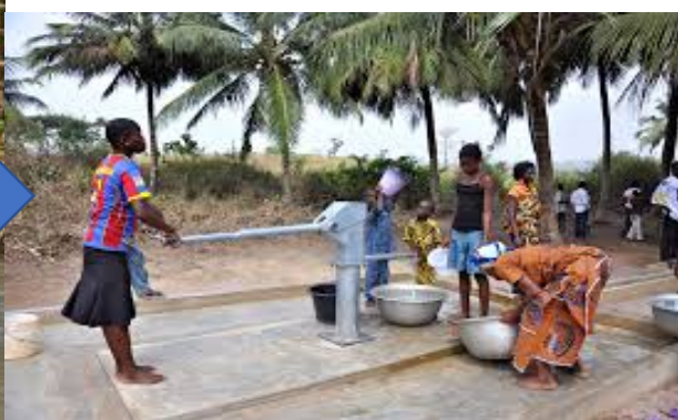
Drilled borehole by 2022
