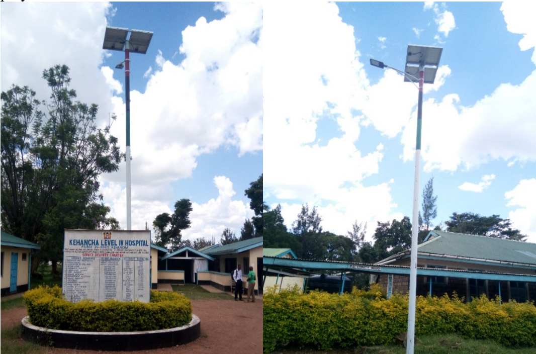
Installed solar lights at kehancha level four
