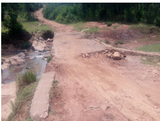
Culvert Road as at 2018 Envisioned bridge by 2022
