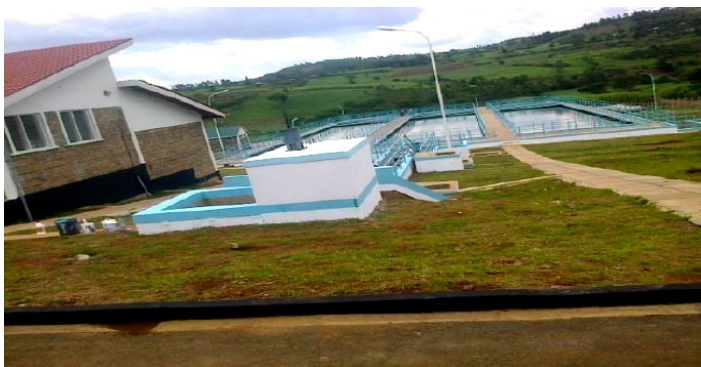
Rehabilitated water treatment system by 2022
