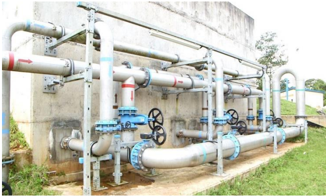
Sand filters with draining pipes
