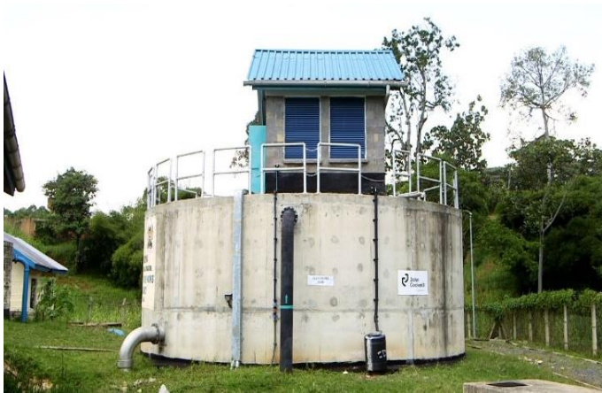
Clear water tank with a dosing unit on top
