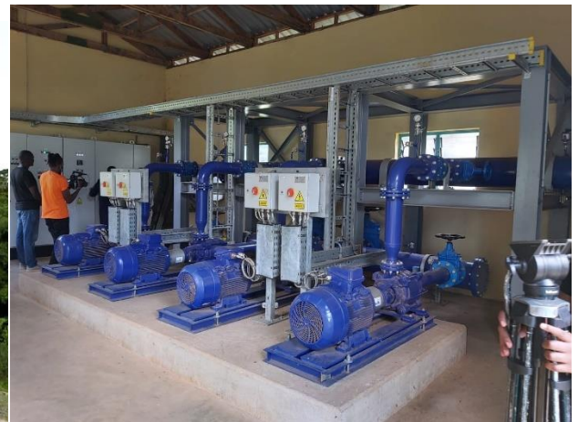
A set of four new pumps connected to hybrid energy supply (solar and electricity)
