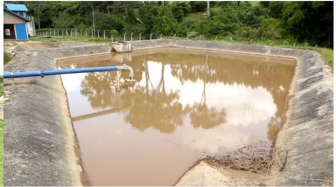
Lagoon for sludge water during water treatment
