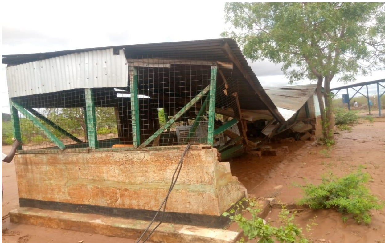
Figure 4: A borehole pump house in Buna, Wajir North, destroyed by the floods
