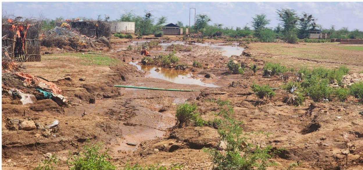
Figure 10: Water piping system exposed and damaged by the floods in Eldas
