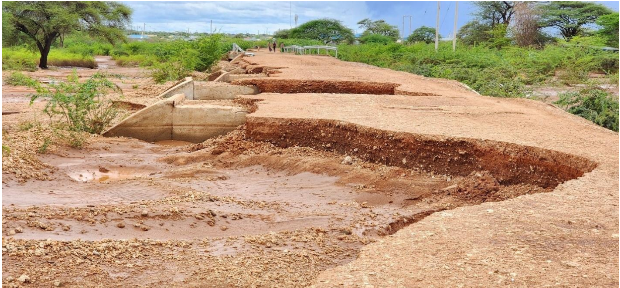
Figure 1: Figure 1 A section of Buna culvert in Wajir North damaged by the floods
