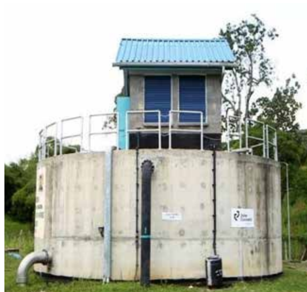
Clear water tank with a dosing unit on top
