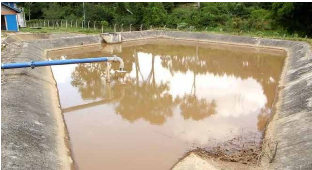
Lagoon for sludge water during water treatment
