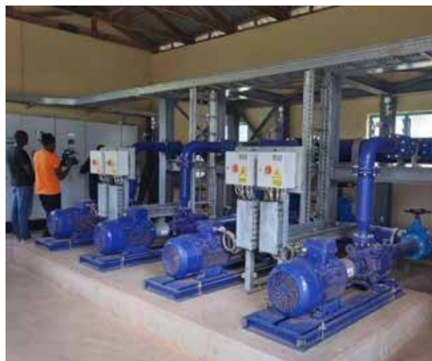
A set of four new pumps connected to hybrid energy supply (solar and electricity)
