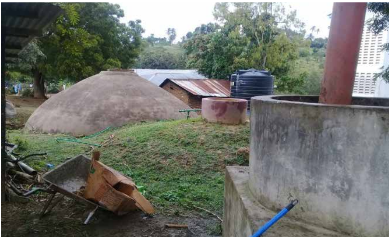
30-meter cubic biogas digester at Malindi High School and Kombeni Girls
