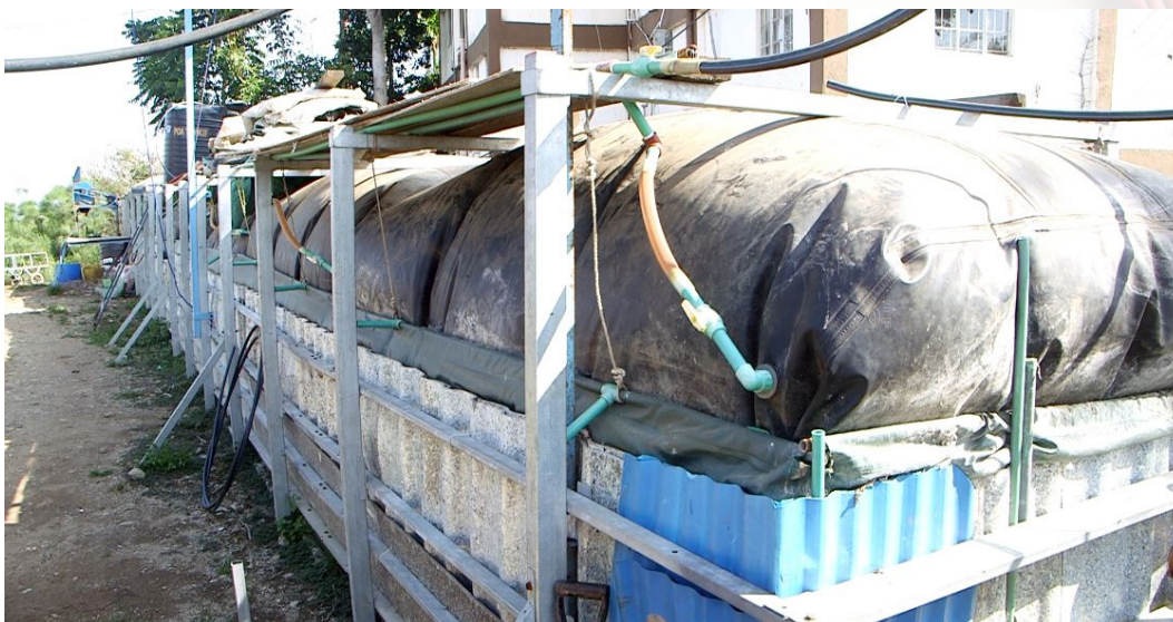
Figure 29: The Bio-digester at Dunga recycling plant in Kisumu County
