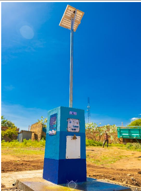
A fully functional solar-powered smart water kiosk
