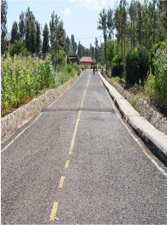
Figure 8: Completed Kabati Road with Markings, Side walk and drainage
