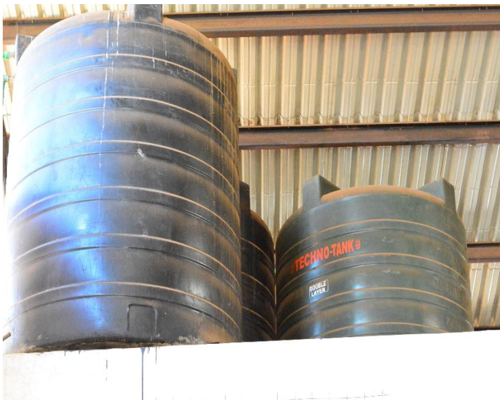
Figure 5: Water tanks for water provision and storage used for cleaning of the market as well as the toilets
