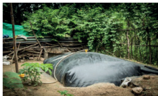
Prefabricated biodigester (price depend on the size (From Kes 80,000 on ward
